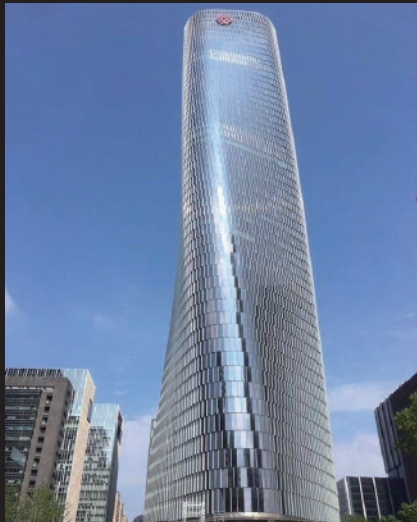
Bank of China Data Center
