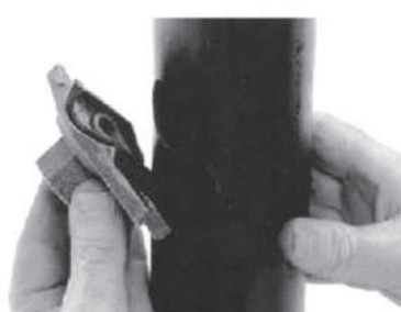
3. Gasket installation
