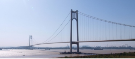
桥梁建设 Bridge Building
