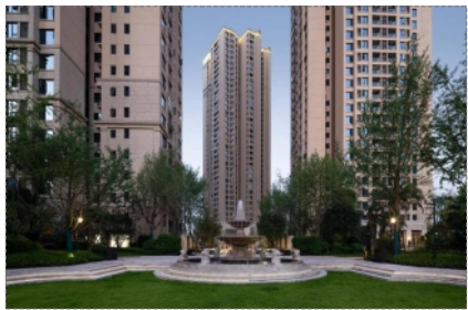
重庆北嘴紫御江山小区 Chongqing Jiangbei District Beizui Royal Purple Jiangshan Residential Areas
