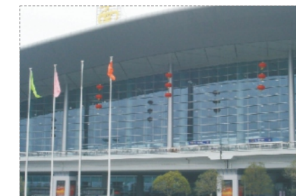
南昌机场 Nanchang Airport
