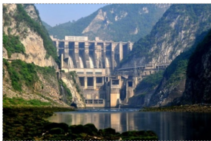
引子渡水电站 Yinzidu Hydropower Station
